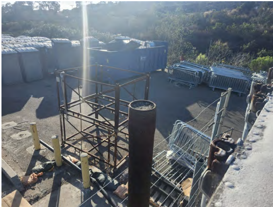
Fig. 4 — 20260716_181136.jpg (~6:11 p.m.). Yard view: rusted steel frame staged on pallets and a loaded roll-off (construction) debris container newly brought onto the site, adjacent to the tank and the property boundary.
