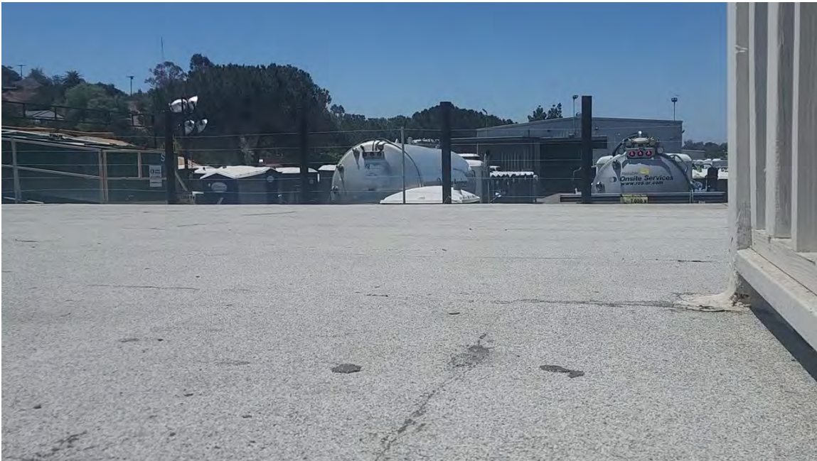
Fig. 6 — “20260802_122031” (≈ 12:20 p.m., August 2, 2026), still from video. A Reliable Onsite Services (“www.ros.ur.com”) bulk-vacuum unit staged directly at the FRAC tank — the most recent capture, one day before this supplement.
