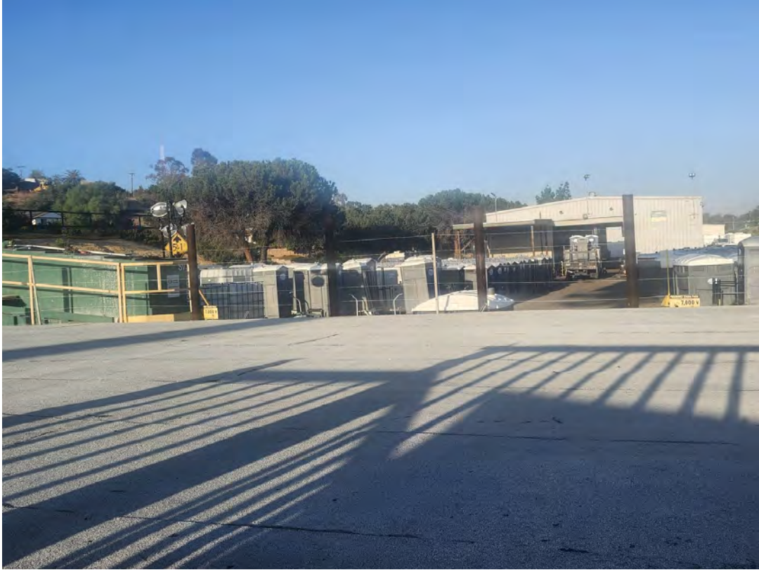
Figure S-1. At approximately 7:07 a.m., July 15, 2026, the vacuum tanker's staging position beside the FRAC-tank enclosure (green, left) is empty — consistent with the ~6:15 a.m. departure I observed and the roughly one-hour absence that followed.
