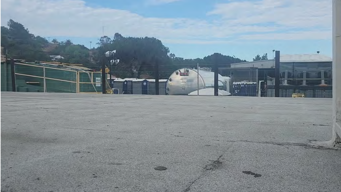
Fig. 1 — “20260720_083302” (≈ 8:33 a.m., July 20, 2026), still from video. The fixed FRAC tank in the operator's yard, with the “7,000 V” bulk-vacuum unit staged at right. July 20, 2026, ≈ 8:33 a.m. clip. YouTube: _____ (insert after upload). Original preserved in NOISE ISSUES\Recordings.
