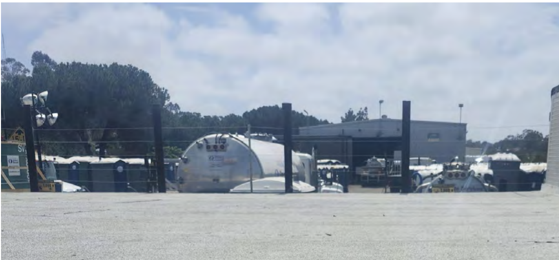
Fig. 17-4 — “20260717_143102.jpg” (≈ 2:31 p.m.). The bulk-septage tanker and service units remain at the tank through the afternoon.
