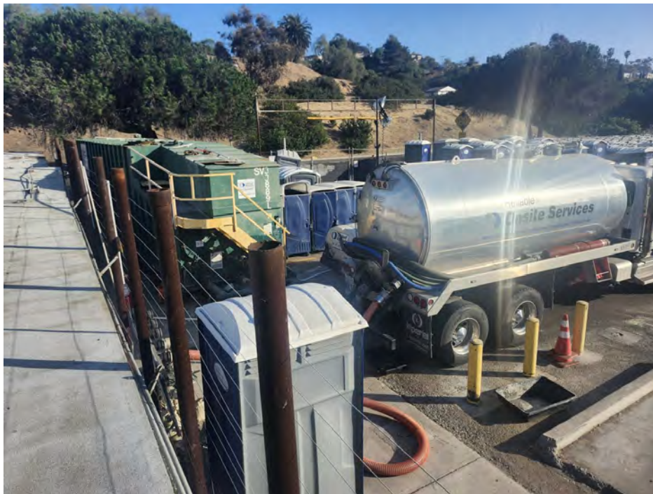
Fig. 3 — 20260716_181152.jpg (~6:11 p.m.). The operator's "Reliable Onsite Services" bulk tanker parked immediately alongside the open FRAC tank, transfer hose deployed; the two operating as one unit, with sandbags staged at the base as apparent secondary containment for spillage.
