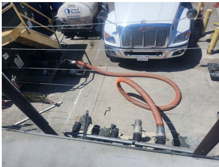
Exhibit 3, Image 124 — August 16, 2026: the BT truck (California plate 95407F4) at the fixed hose and manifold serving the FRAC tank.
